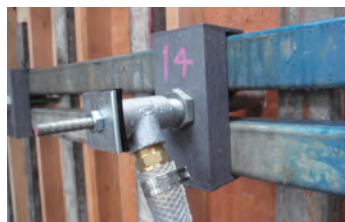
Photo-3 Combined Separator and Cooling Water Inlet
