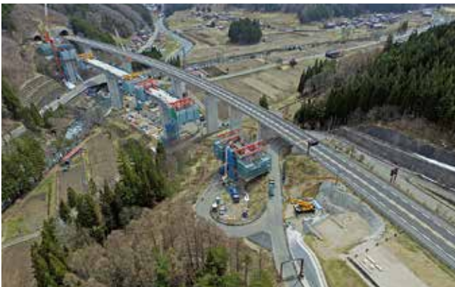
Figure-3 Sounori Bridge construction progress
