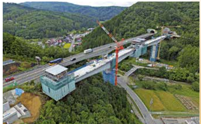
Figure-4 Kurotani Bridge construction progress
